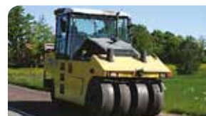
Rolling of surface dressing/chipseal.
