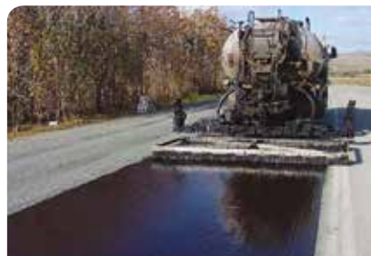
Scrub seal: Broom dragged behind bitumen distributor pushes binder into cracks.
