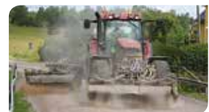
Sweeping of surface dressing/chipseal.
