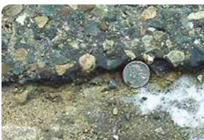
Otta seal after trafficking. Soft binder has migrated to the seal surface.
